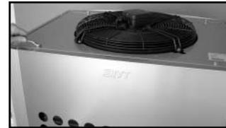
Remove the covers by loosening the screws on top of the heat pump.
