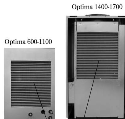
Clean the dirt from the coil fins using a degreasing agent and water.
